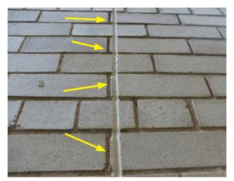
Photo 2 Poorly Aligned Remedial Expansion Joint
