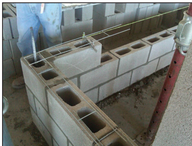
Figure 1 - Ladder type joint reinforcement laid dry on the masonry units
