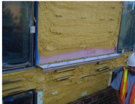
FIG. 6 XPS used in conjunction with SPF to protect the self-adhered membrane.
