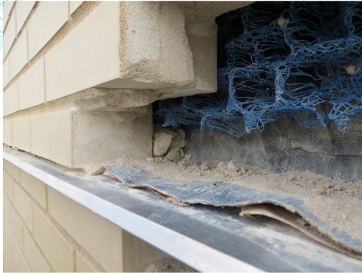
Self-adhering membrane flashing without backing paper removed
